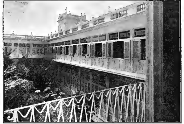
REAR VIEW OF THE BUILDING.
